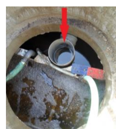
Fig 5: Sampling Tee fitting inside an Oxyfix® C-90 5 EP Unit
