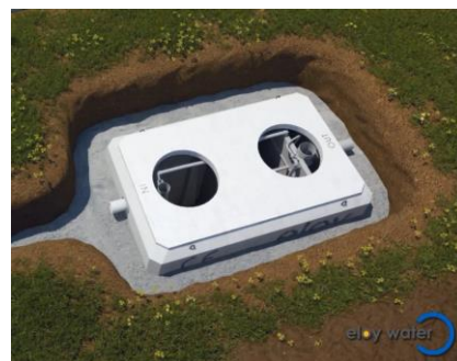
Fig-15: Compact backfill
