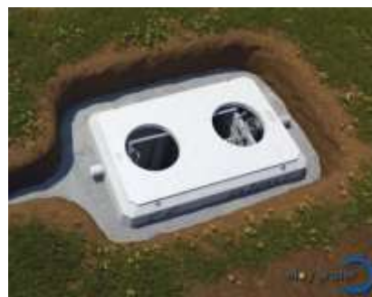
Fig-21: Compact backfill
