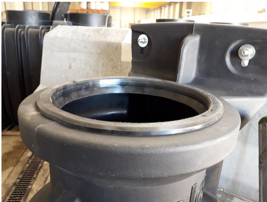
Fig.14 – installation du joint Ø315mm
