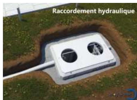
Fig-24 : Raccordement hydraulique
